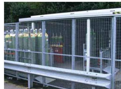
Figure 7: Fence protecting gas bottles Source: Suva
